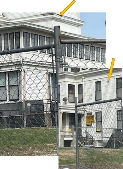
The exterior of the property is damaged. The roof is missing shingles, and the gutters are falling off, the paint is peeling, and the stairs are not operational.
