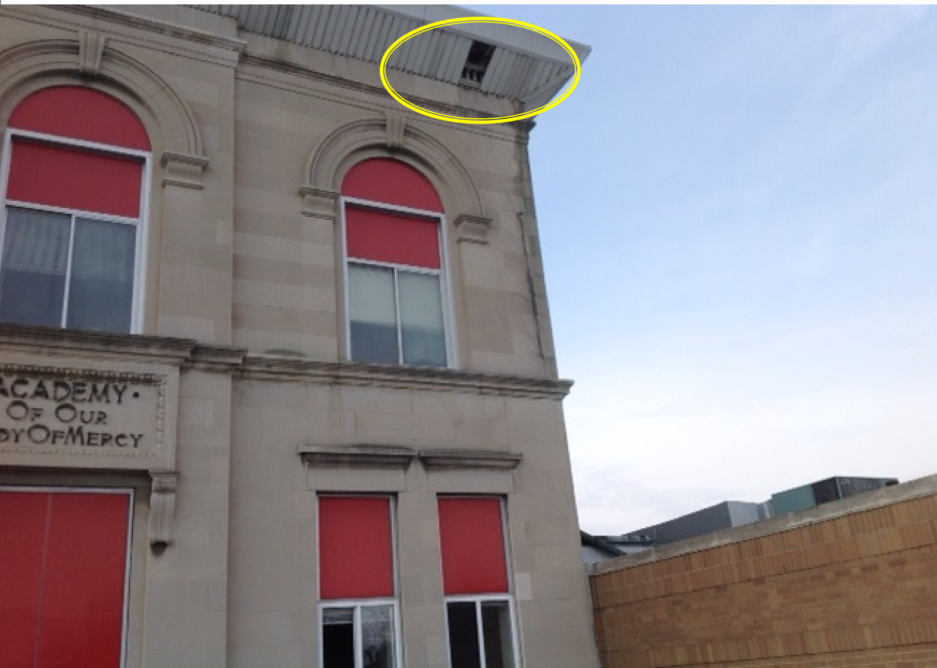
View of damaged soffit.
